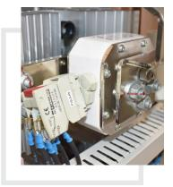
Additional diode in each branch in order to provide full performance after failure of one diode in each branch.
